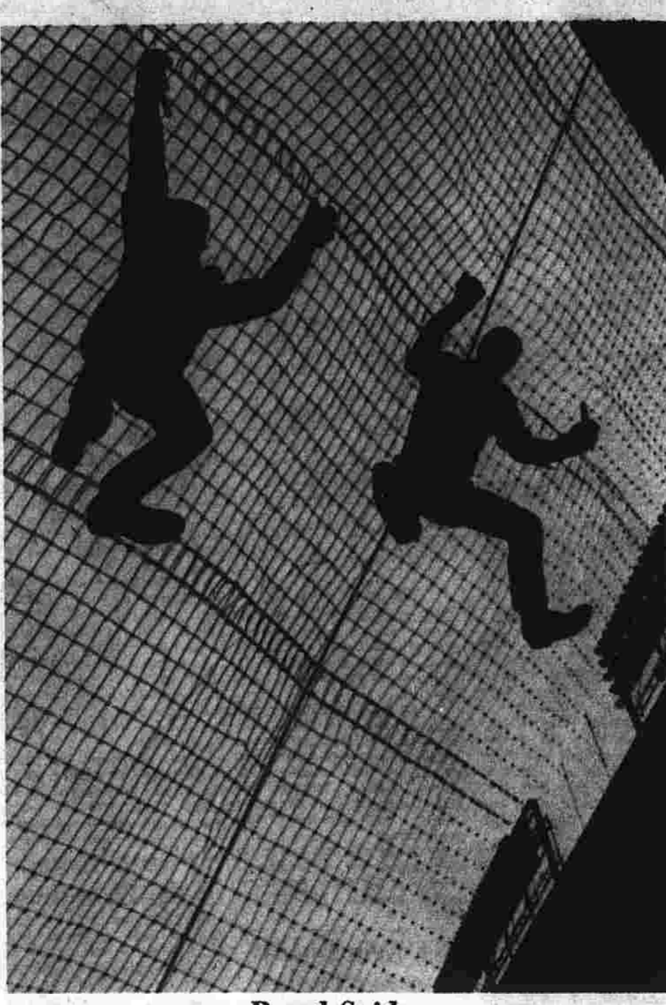
Workers climb the steel screen behind home plate at Kansas City Municipal Stadium to prepare for another baseball season for the Royals. (AP photo)
